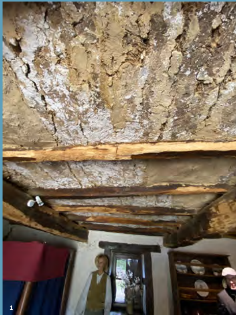
1. Details of the cob ceiling in farmhouse no. 10 on the Acadian Line
